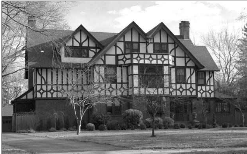
Appropriate Landscaping and Site Maintenance on a Tudor Property on Prospect Avenue
