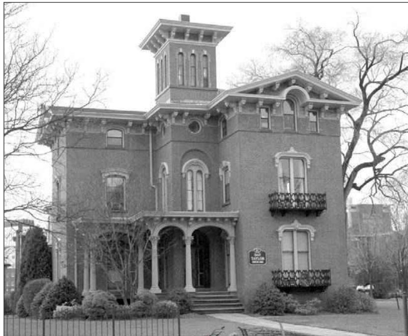
The Wrought Iron Fence Surrounding this Italian Villa on Wethersfield Ave is a Character-Defining Feature.
